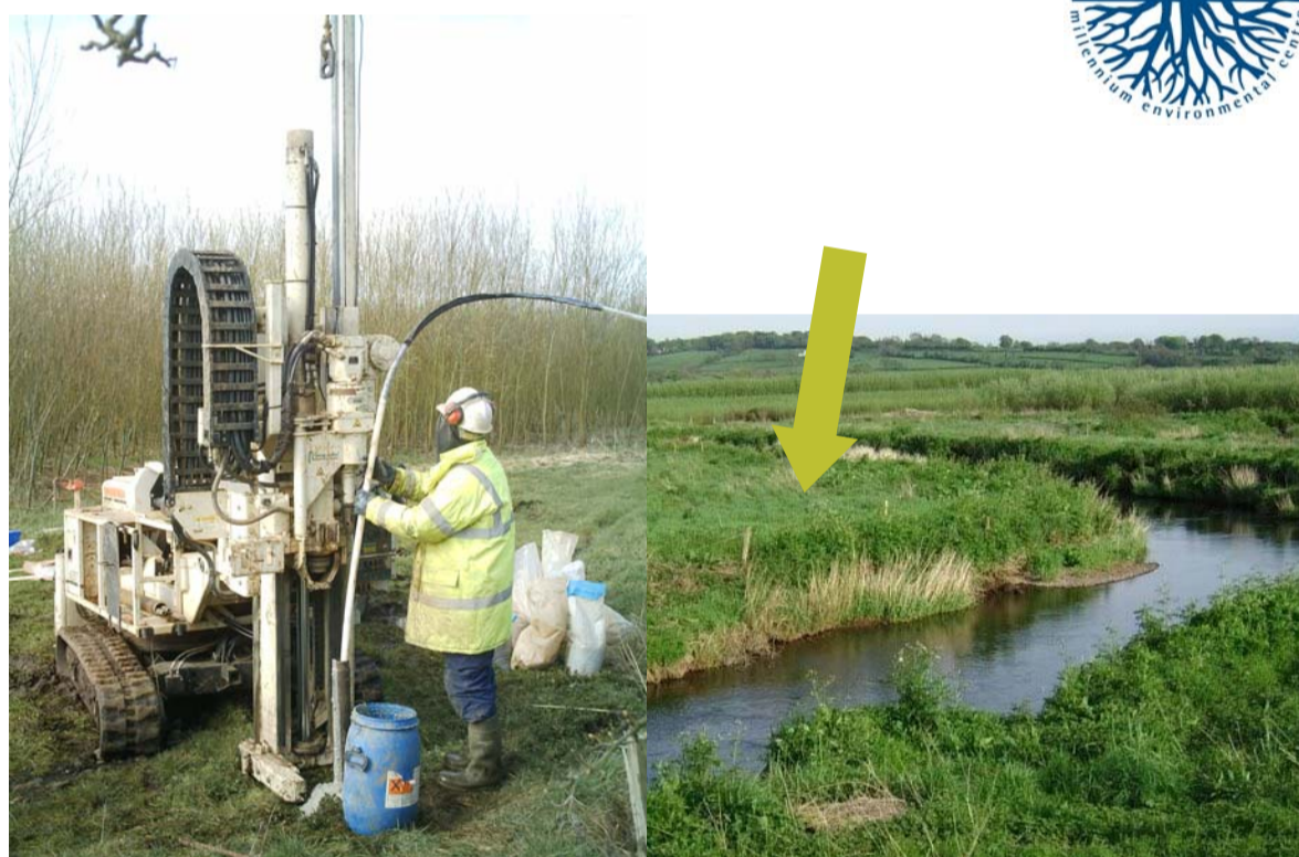
Installation of a monitoring borehole network at the ecos centre
