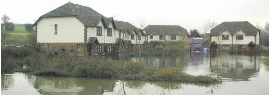
Groundwater flooding in 2000, in Farringdon, Hampshire (Jacobs, 2006)
